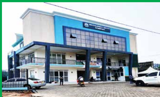
The New Arua commercial complex housing WSACCO Arua branch
